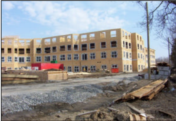
A look at the construction site: Phase 3
