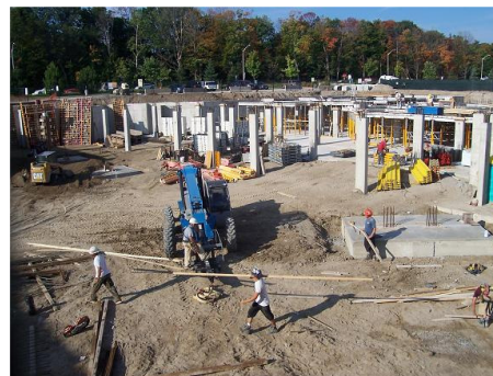
Work on the parking garage is progressing
